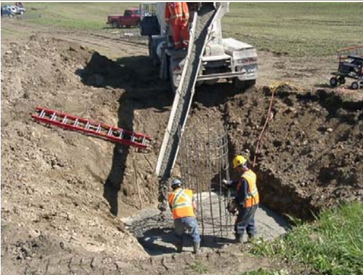
Construction of wind turbine foundation
