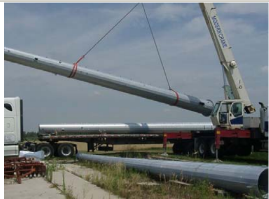
Arrival of wind turbines and towers
