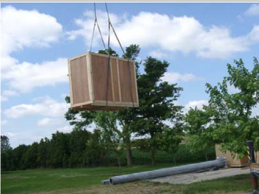
Arrival of wind turbines and towers
