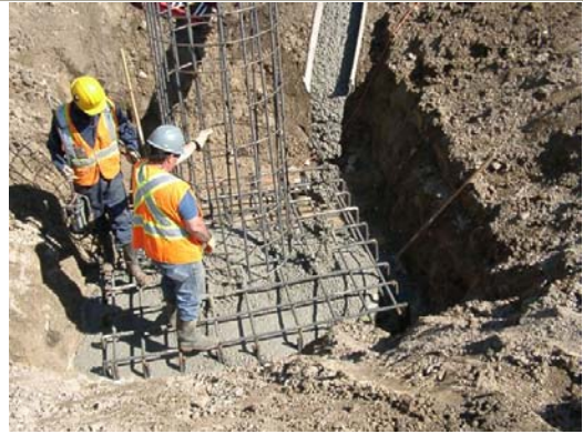
Construction of wind turbine foundation
